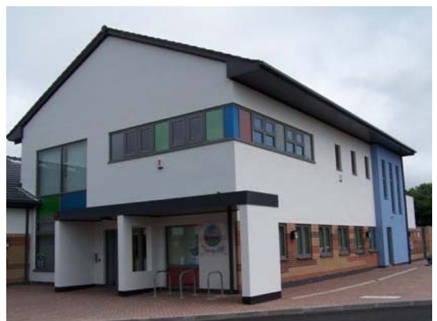
Plym Bridge House, Child & Adolescent Mental Health facility
